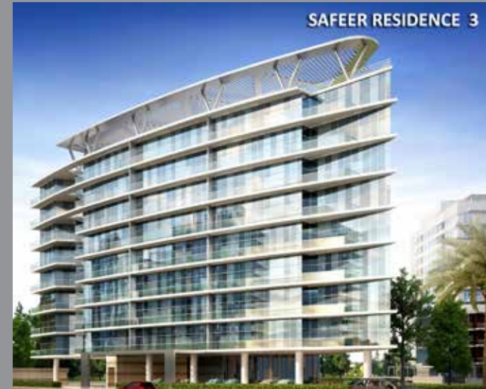
SAFEER RESIDENCE-3 Dubai Land Residence Complex
