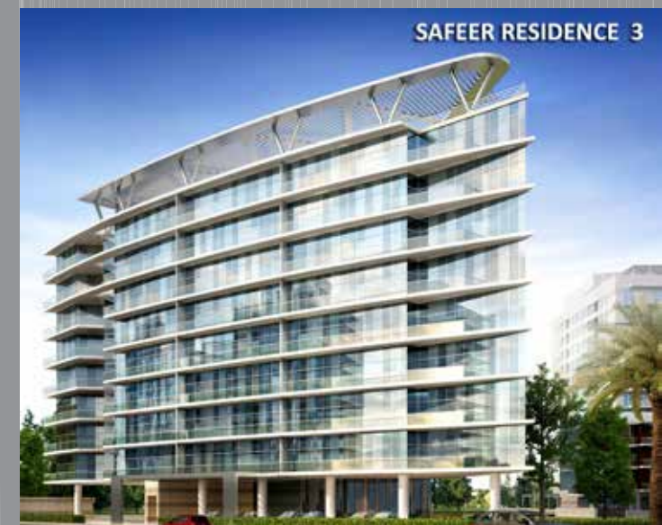
SAFEER RESIDENCE-3 Dubai Land Residence Complex
