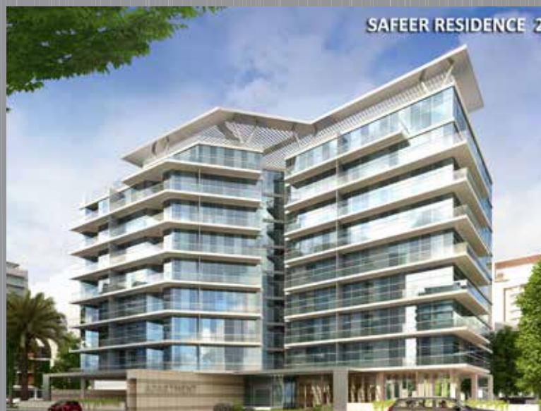
SAFEER RESIDENCE-2 Dubai Land Residence Complex
